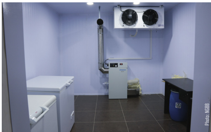
The completed dry room with freezers, Munters dehumidifier, cooling unit and blue drum drying kit.
