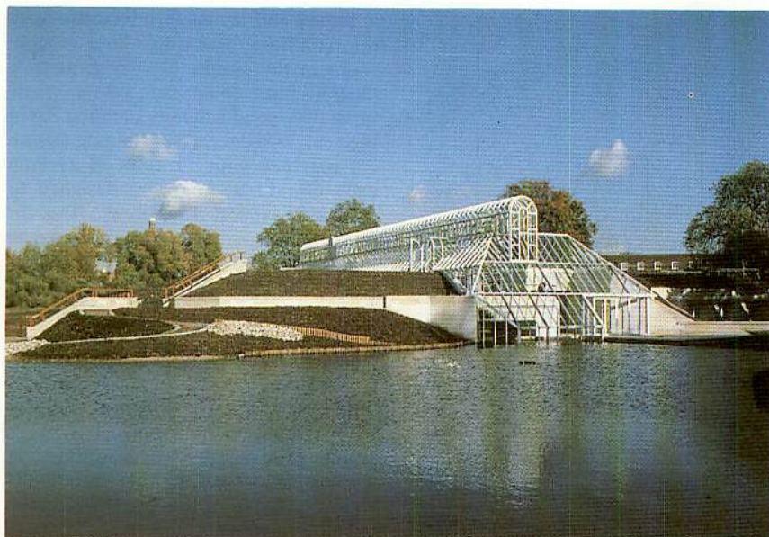
Figure 2 The new Sir Joseph Banks Centre, showing the public entrance and the central glasshouse, which will house live plants, with the exhibition hall to the left. (Photo: Royal Botanic Gardens, Kew).
